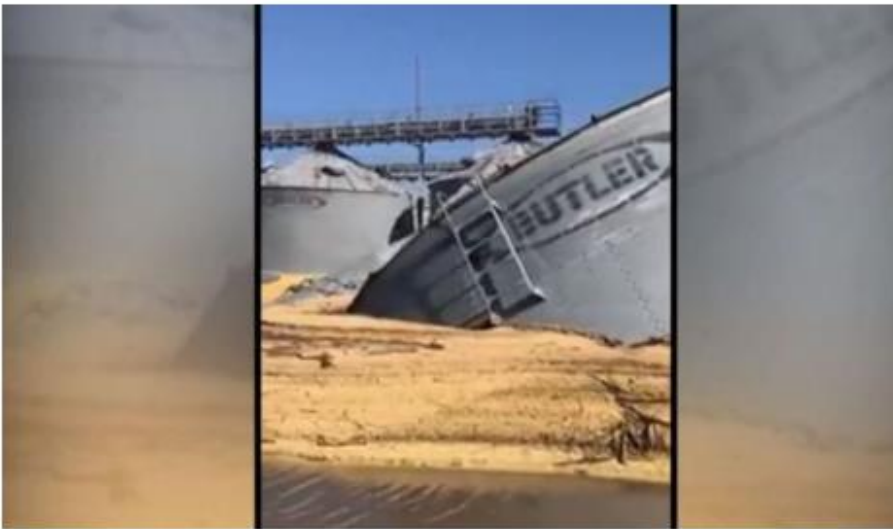
US grain bins collapse under catastrophic Iowa floods. via Youtube video
