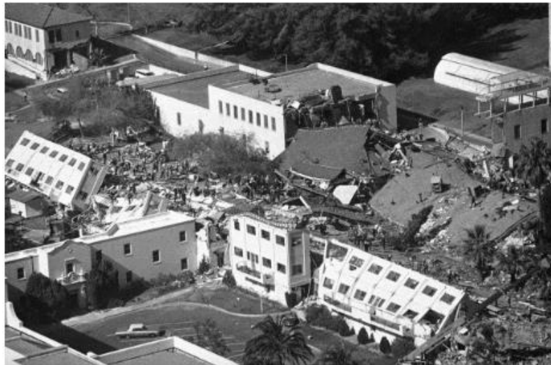
Damage at the San Fernando Veterans Administration hospital in Sylmar killed 49 people. Photo by Orange County Register.
