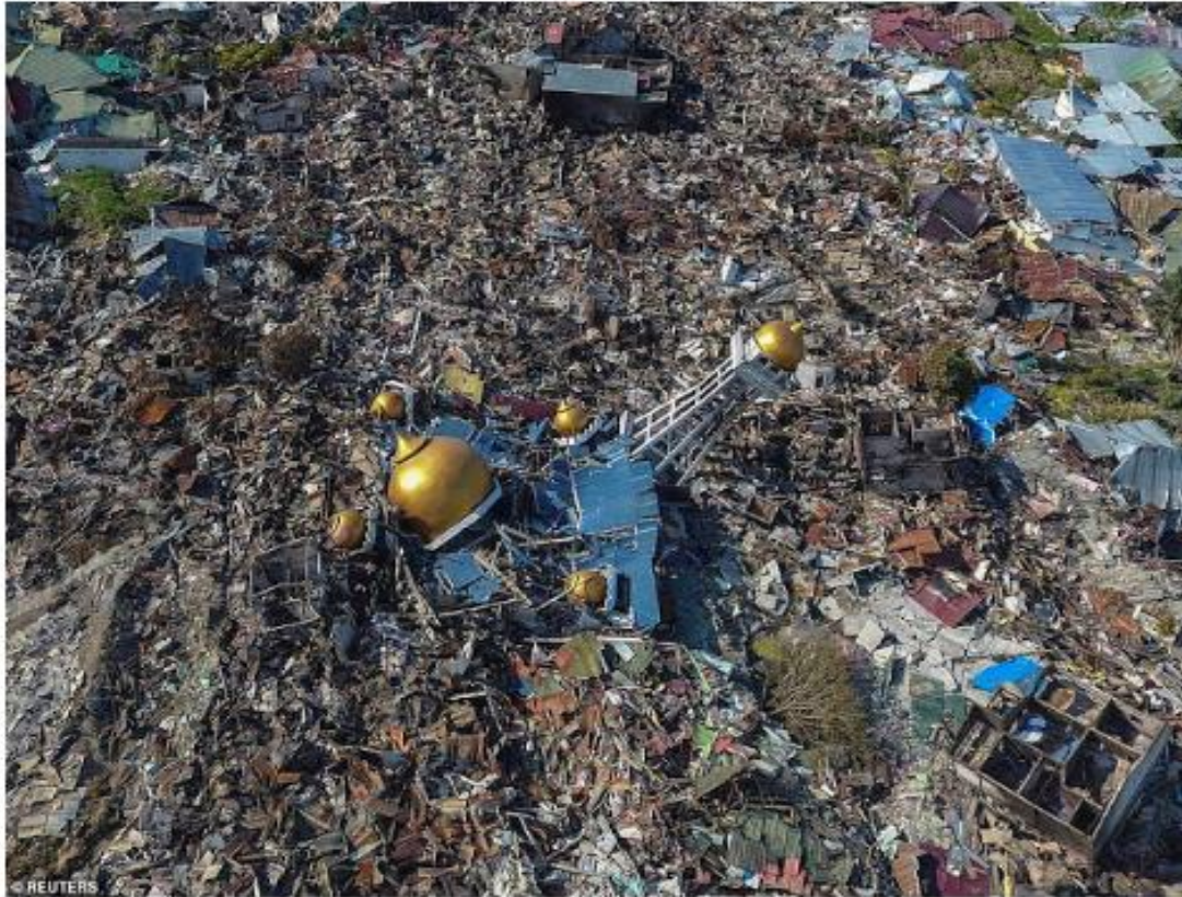
An aerial view of an area devastated by an earthquake in Palu, Central Sulawesi, Indonesia. Photo credit Daily Mail
