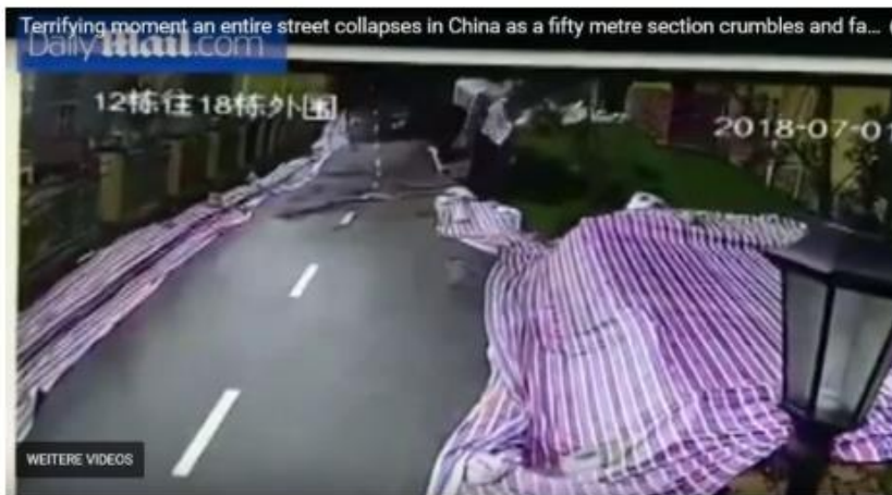
Terrifying footage has emerged of the moment a fifty-metre section of a major road collapses in China.
