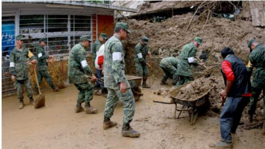
Mexican soldiers help dig out damaged homes in Veracruz, Mexico after they were buried by landslides triggered by Tropical Storm Earl on August 6, 2016.
