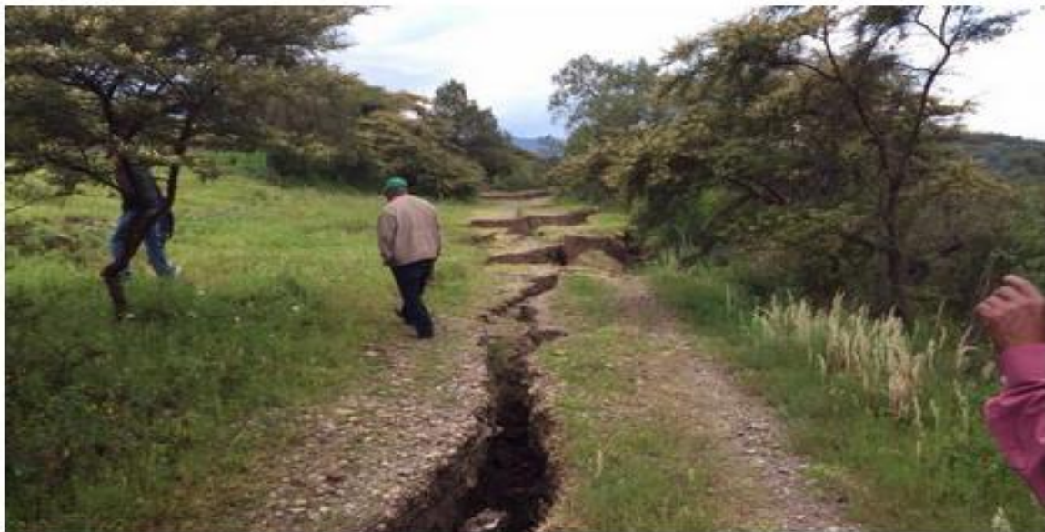
Photo of the giant crack forming in the district of Oaxaca, Mexico
