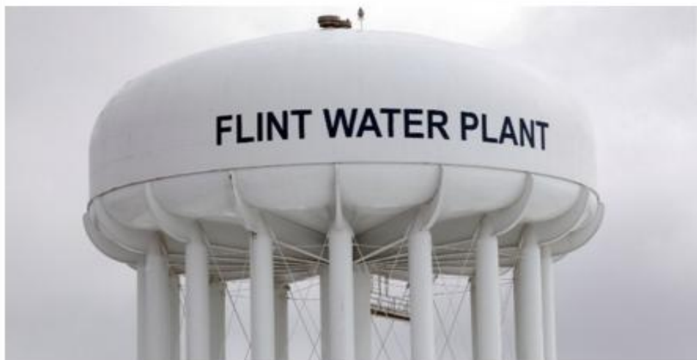
The Flint Water Plant tower.
