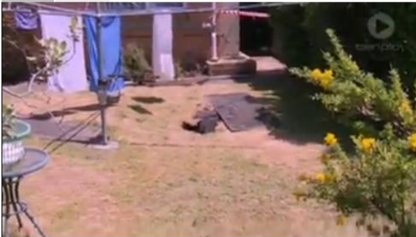
Woman falls into 3 metre sinkhole
